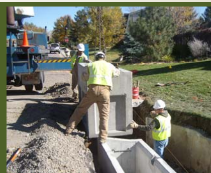
Easter/Verbena Infrastructure Project
